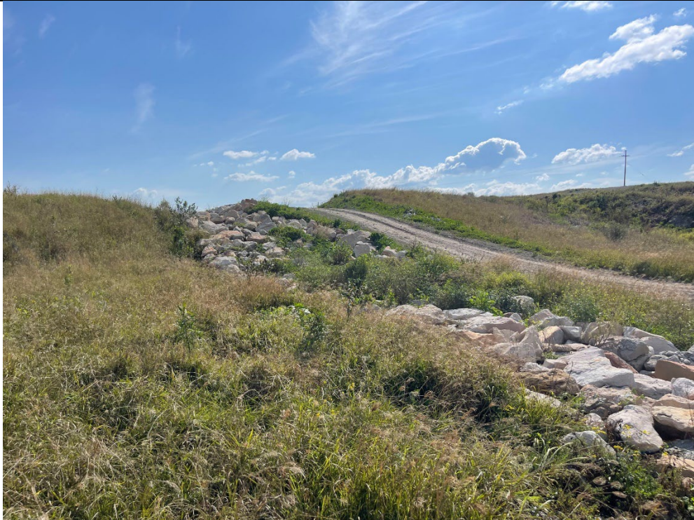
Photo 20 Riprap used at surface water spillway to Stage 2 leachate dam
