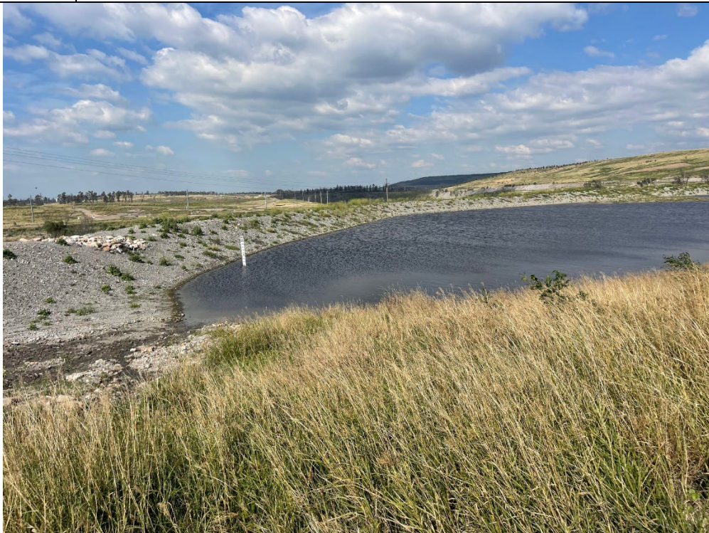
Photo 21 Stage 2 leachate dam, showing water level marker and EPL discharge point to the left side, identified via rip rap on bank.
