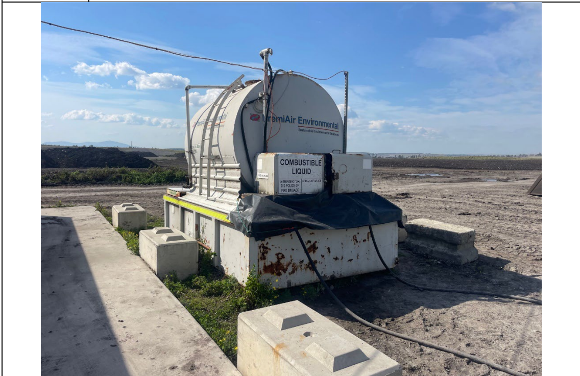
Photo 9 Diesel above ground storage tank, drip trays covered in plastic to prevent rain water build. No visual evidence of spills or leaks.
